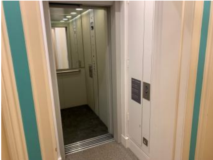
Lift to all floors in the manor house
